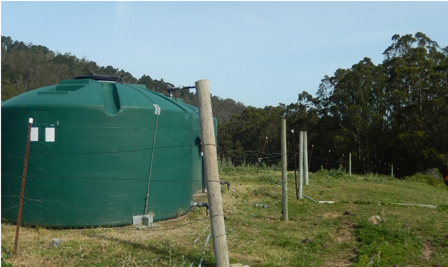
View 4. View of the project area looking north from the existing water tanks.
