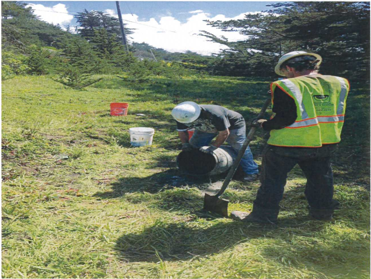
Grouting test bore hole B2
