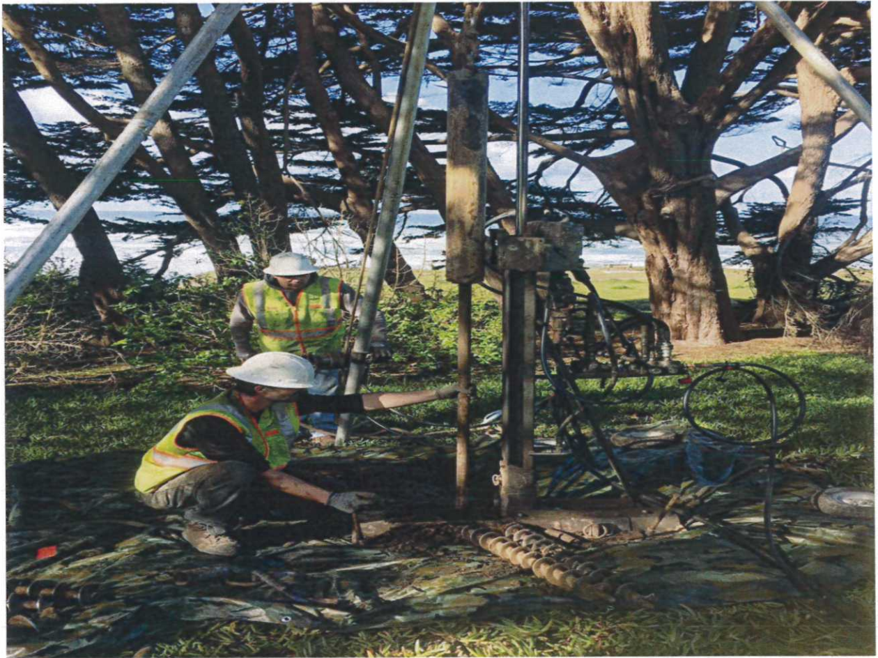
Drilling operations at test bore hole B1
