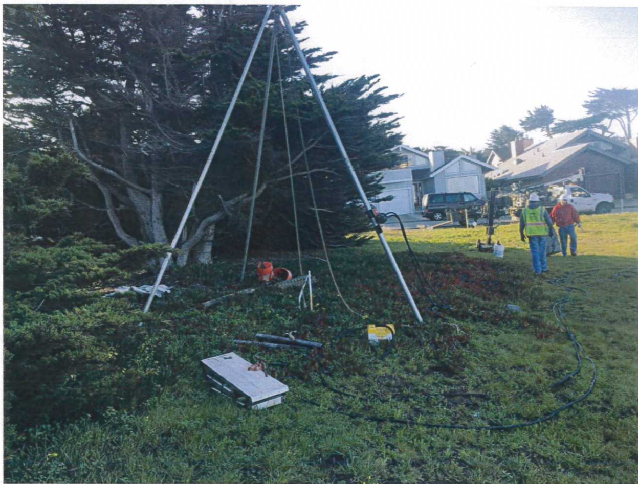
Drill setup test bore hole B4
