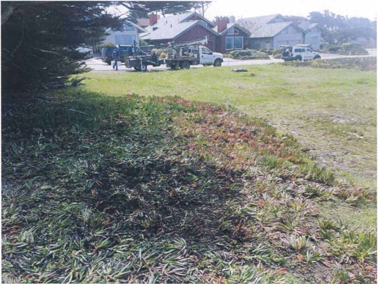
Ground surface after drilling operation test bore hole B4
