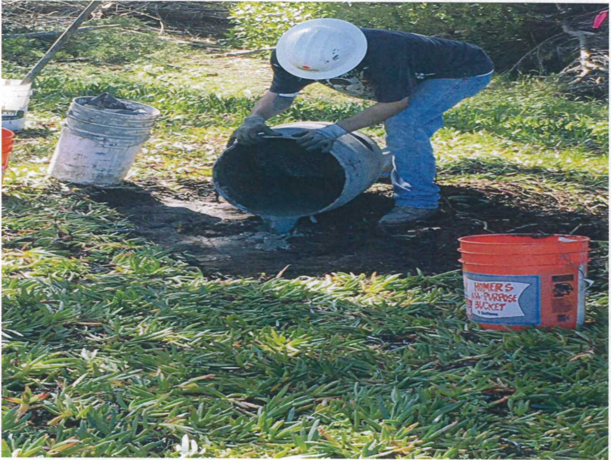
Grouting of test bore hole B1
