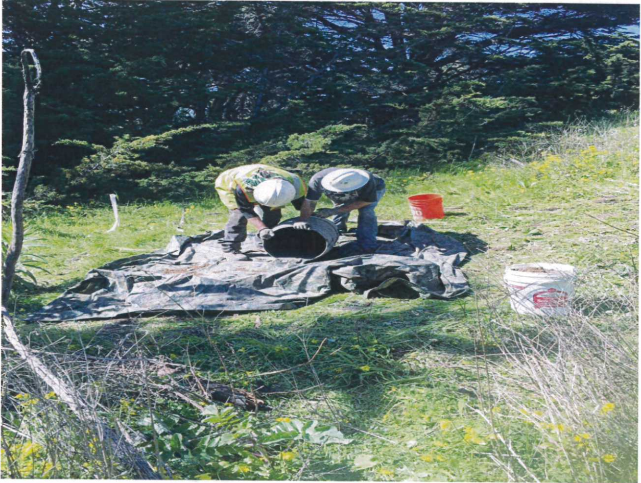
Grouting of test bore hole B3
