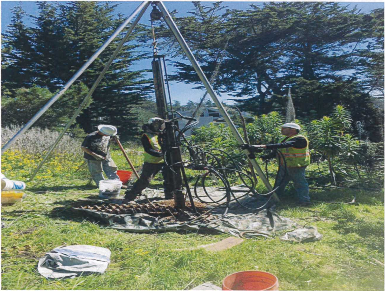
Drilling operation test bore hole B2
