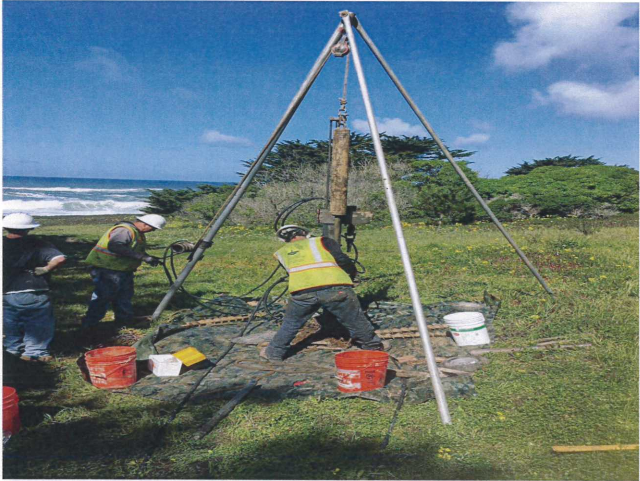
Drilling operation test bore hole B5
