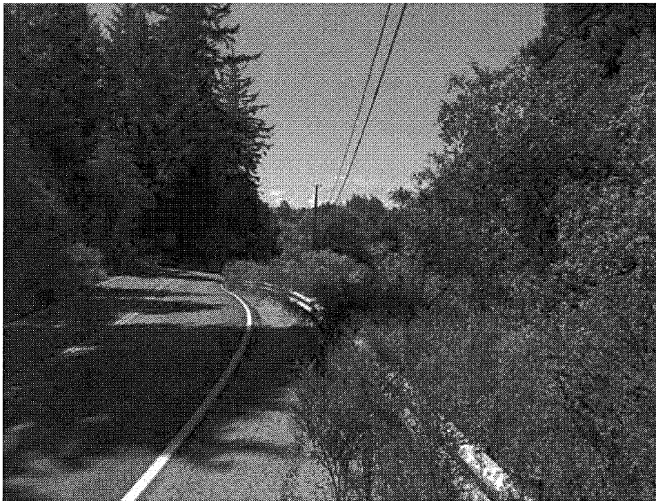
Photograph 6 View south of proposed Node 057A site.
