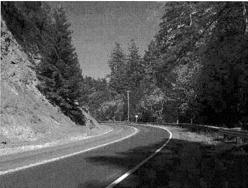
Photo 4: Node 049A Area Overview (East Northeast)
