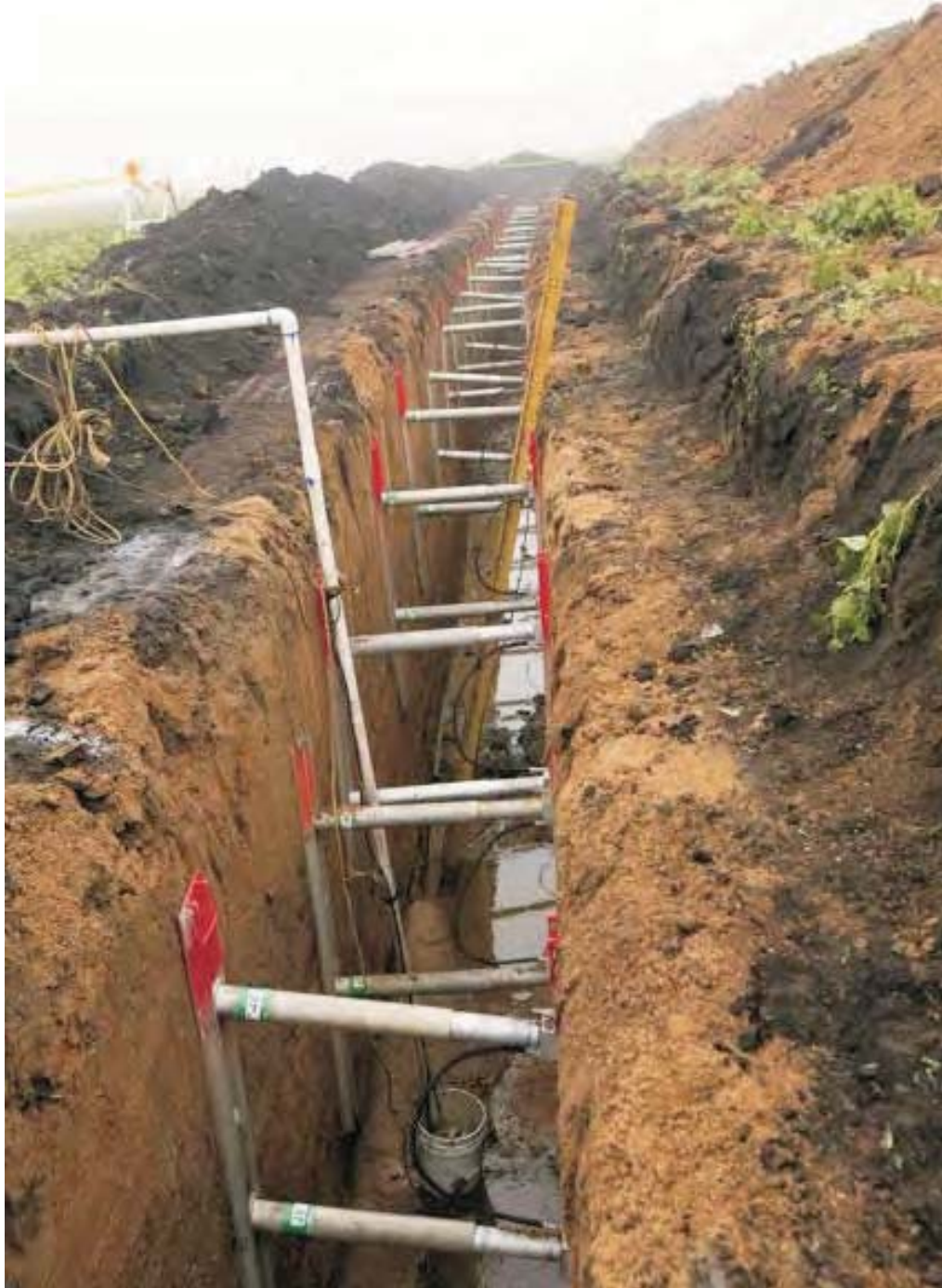
View of Trench B, from West End
