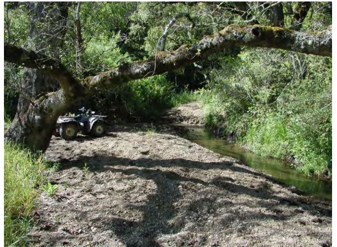
MP 19: Ford crossing over Harrington Creek.
