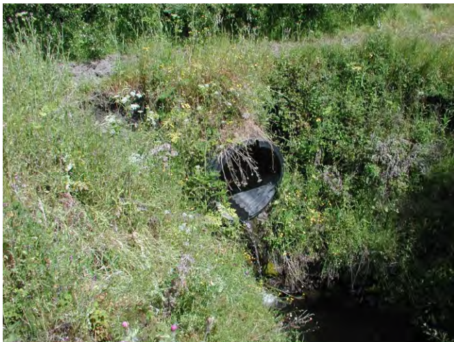
MP 57: Culvert outlet
