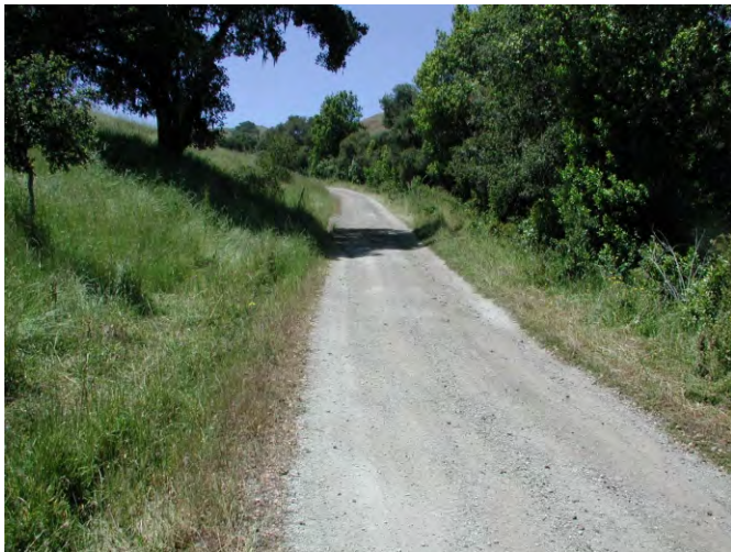
MP 14: Long inboard ditch
