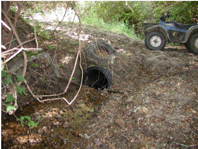
MP 18: 24" culvert on infrequently used tractor trail
