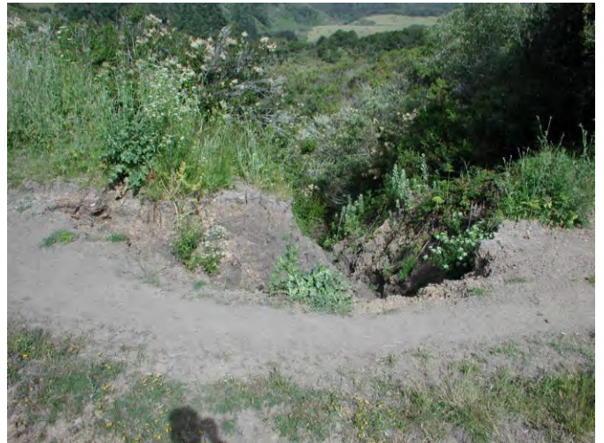
MP46: Gully narrowing road.
