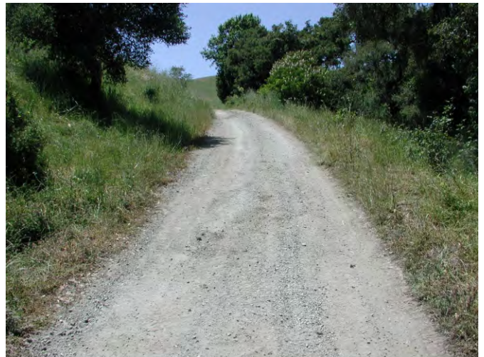
MP 15: Long inboard ditch
