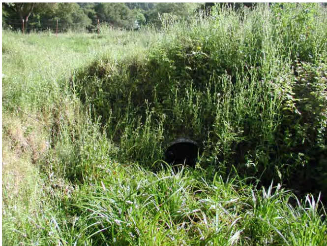
MP 38: Inlet to culvert
