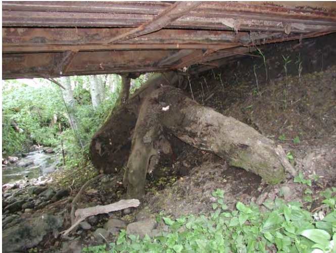
MP 12: Looking at right bank abutment of railcar bridge
