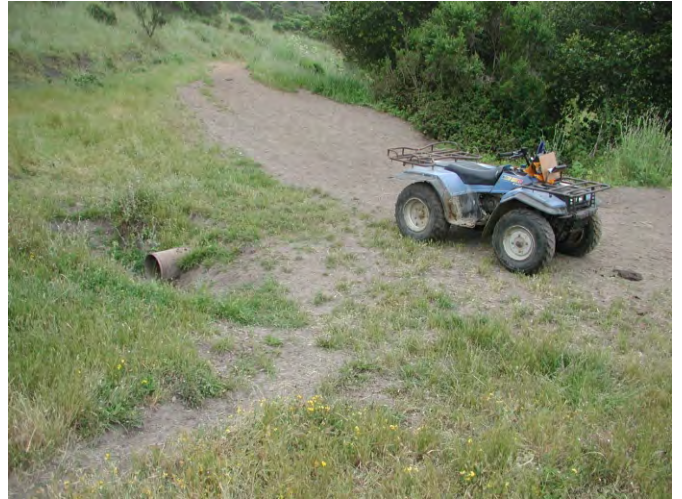
MP 45: Culvert inlet
