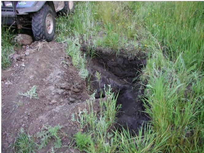
MP 26: Hole in road needing to be backfilled
