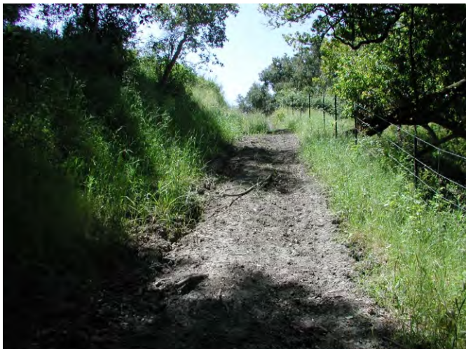
MP 28: Steep road reach leading to culvert
