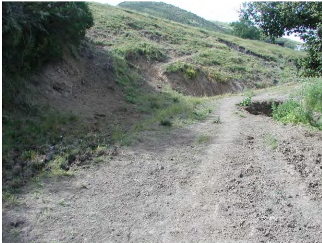
MP 46: General site photo
