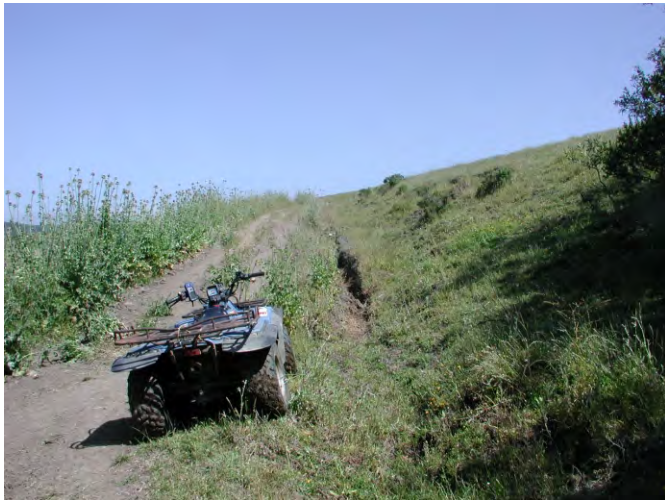
MP 48: Looking up eroding road
