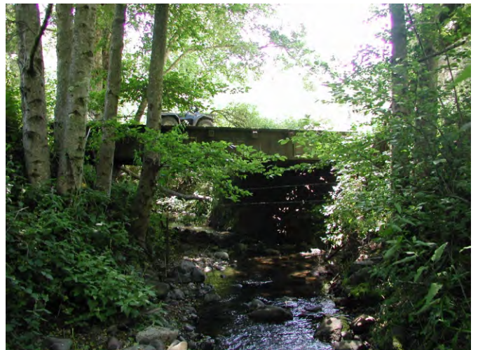
MP 12: Rail car bridge over Harrington Creek.
