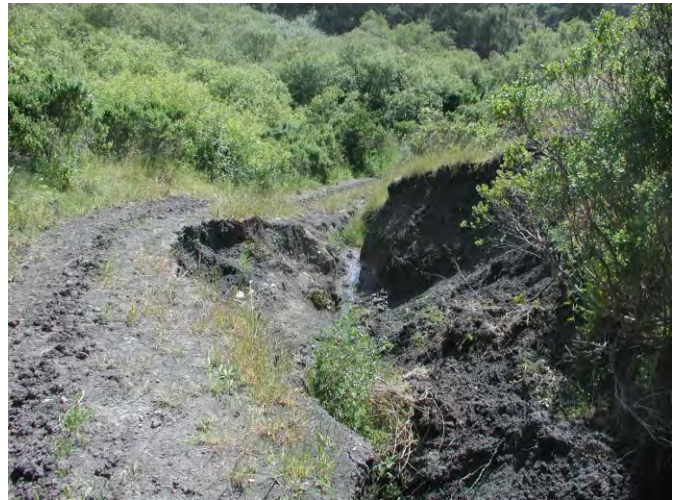
MP 55: Looking down lower gully
