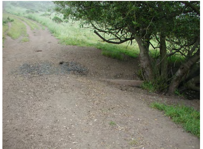
MP 42: Culvert outlet
