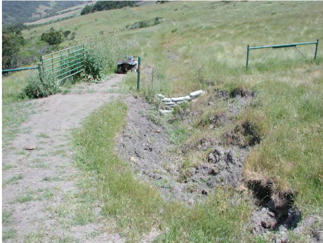
MP 50: Concrete sack headwall used to curb ditch
