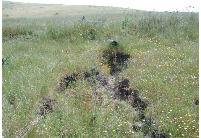
MP 50: Gully at outlet of culvert
