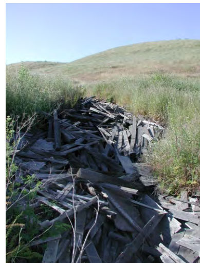
MP 21: Gully armored with wood.
