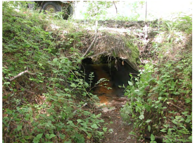
MP 28: Inlet to culvert
