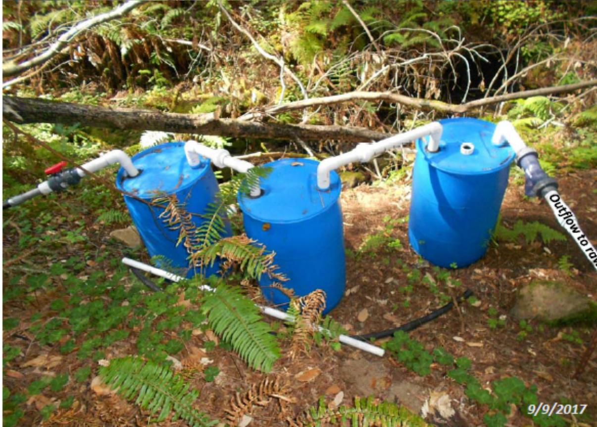
**Figure 1. Existing diversion structure on Hoffman Creek, Redwood Glen, San Mateo County, CA.** The diversion structure consists of a stainless-steel sink attached to a redwood log across this creek. Sediment entrained in the line extending from the sink to the raw-water tank accumulates in a series of three 55-gallon drums used for settling. Water and sediment is flushed onto the bank during maintenance twice a year.
