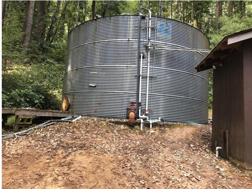
**Photo 3.** The 70,000-gallon raw water storage tank.
