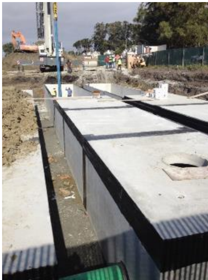
Figure 2. Construction of the Wet Weather Storage Facility on Burnham Strip in 2012
